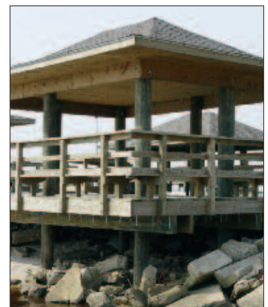
Round timber piling – marine application
